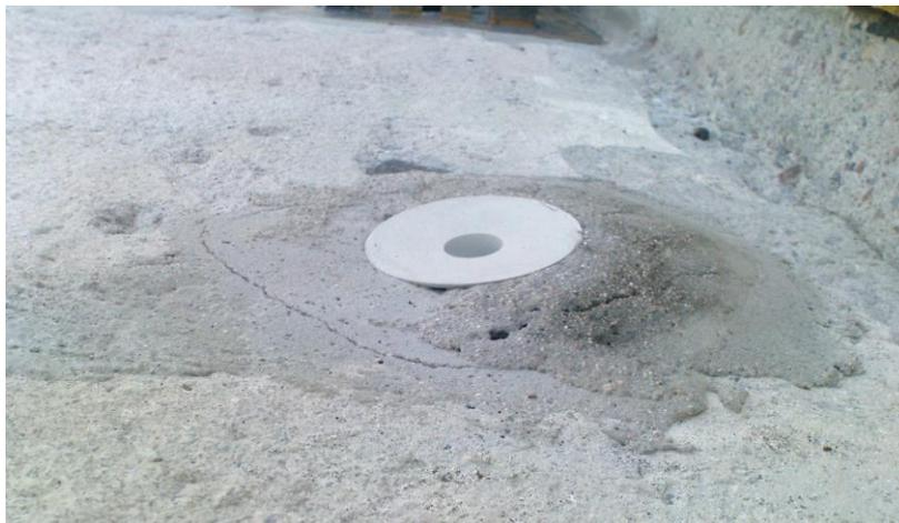
Figure 4: Concrete surface not suitable for installation of waterproofing (Photo: Mikael Kinnmark, DAB Domiflex AB)
